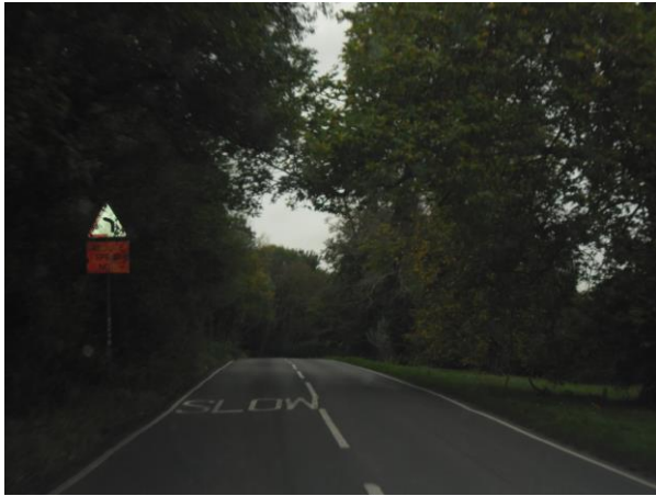
Image 3 – View travelling northbound on Coopersale Street before bend. Bend warning sign is in poor condition.
